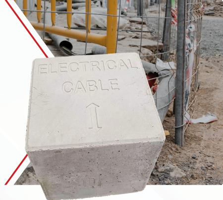
Electrical and Telecommunications Route Markers are essential in the management and maintenance of infrastructure, specifically electrical and telecommunications. Follow safety protocols and mitigate risk with the markers placed above or near underground utility lines to provide critical information to workers, excavators, and other stakeholders.
