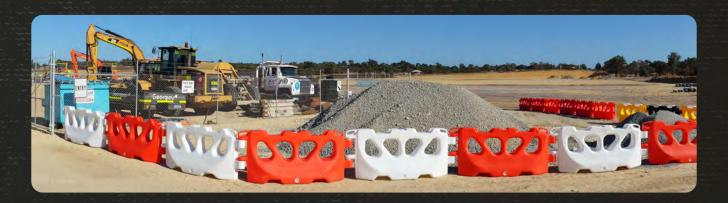
Rounded corners make it safe and easy for workers to handle, and a simple interlocking pin and hole system is moulded into each barrier module, resulting in a one-piece unit with no loose pins. Built-in handles help with the interlocking process and carrying the barrier when empty.
