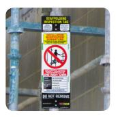
Fix MAXSafe® Scaffold tag to the most visible place on scaffold and access will be clearly and concisely prohibited while installation is in progress.
