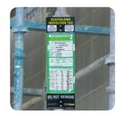
For Certification of Scaffold, simply fold tag to next stage and clip in tabs to show that the scaffold has been certified and can be accessed.
