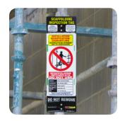
For dismantling or modification, simply fold tag back to Step 1, which will alert all users that the scaffold may not be accessed. (The tag does not have to be removed to fold back.)
